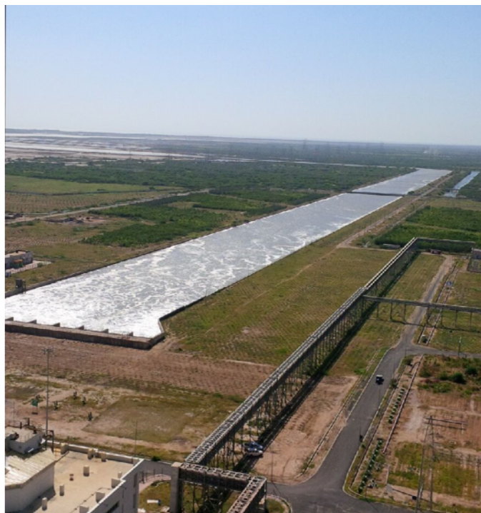
Figure 3: Outfall channel taking water from the plant to the sea
