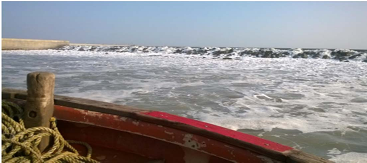
Figure 4: Warm water from the outflow discharging over the weir to the marine environment
